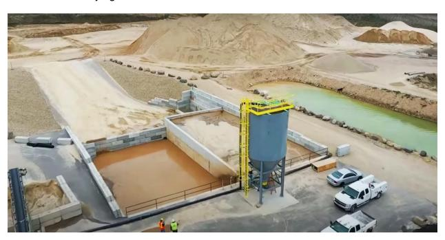
Clearwater worked with Tri-County to redesign their process water flow path to include: a slurry tank, CW1400HC, M500PP, AutoFloc Dosing System, two mud cells with sump.
