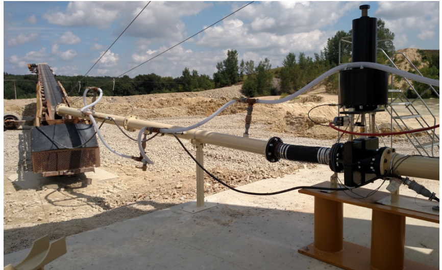
Material is automatically dosed with flocculants again when it enters the discharge pipe, before being conveyed to a containment area.
