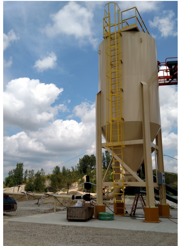
Wendling operates a single 13,000-gal. clarification tank where flocculant is added via an automated system.
